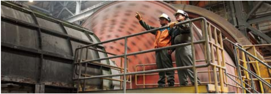
Collahuasi's concentrator plant
